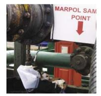
Fuel oil sampling is an essential element of any bunkering operation.
